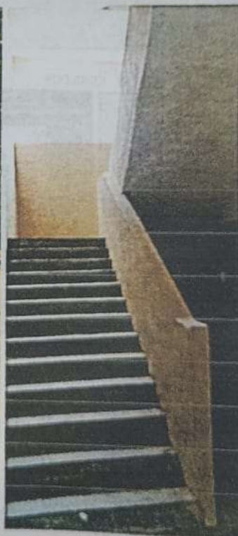
VIEW OF STAIRCASE
