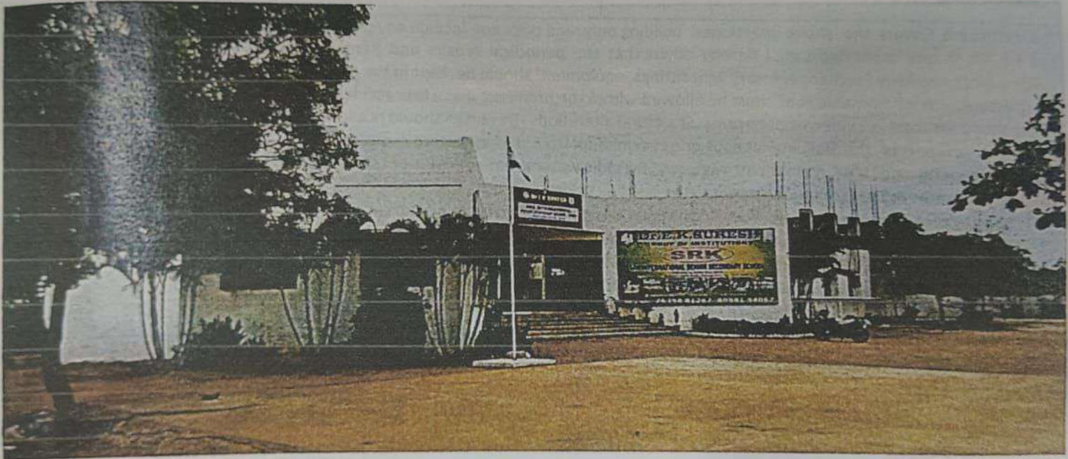
PHOTO SHOWING THE FRONT ELEVATION OF SRK INTERNATIONAL SENIOR SECONDARY SCHOOL, AYEET MAIN ROAD, R.No 4/27, KEEZHUR VILLAGE, KURINJIPADI TALUK CUDDALORE DISTRICT -607302
