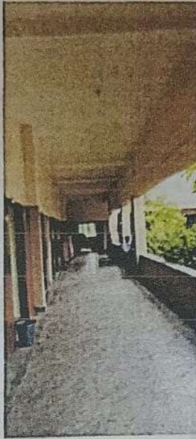
VIEW OF CORRIDOR
